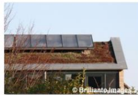
green roof solar hot water panel -Schönberg Germany (C) Brilianto.JPG
